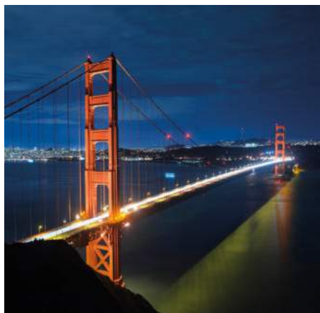
GOLDEN GATE BRIDGE
